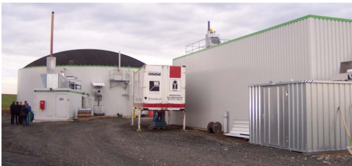
Figure 35: Biogas installation with two digesters (continuously flow type on the left and pug flow type container on the right) in Germany
